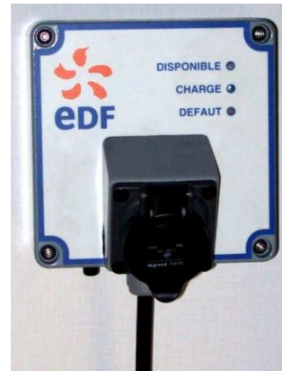
Figure 9: Simple charging plug in metal box destined to be used in parking areas that are accessible to the public
